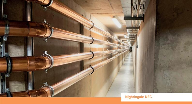
"It was our responsibility to deliver the infrastructure that would carry the medical oxygen and air around the NEC Nightingale, a massive operation that involved two 108mm ring mains, each 3km long, together with another 12 km of 54, 35 and 15mm pipework."
