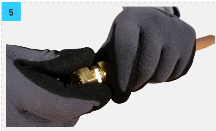
5. Hand tighten the nut onto the fitting.
